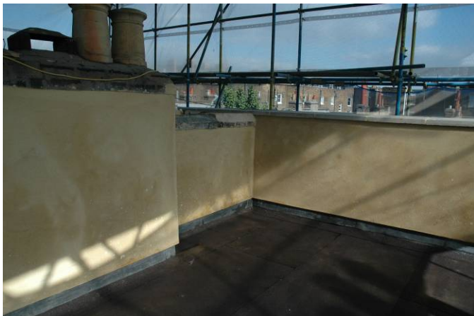
External: Photos (a) & (b) Completed rendering at roof level
