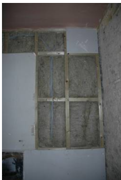
Internal: Photos (a) & (b) Sound insulation (c) Studwork in 2 nd floor flat (hallway outside bedrooms) and (d) insulation, wiring and pipework in the 1 st floor ceiling.
