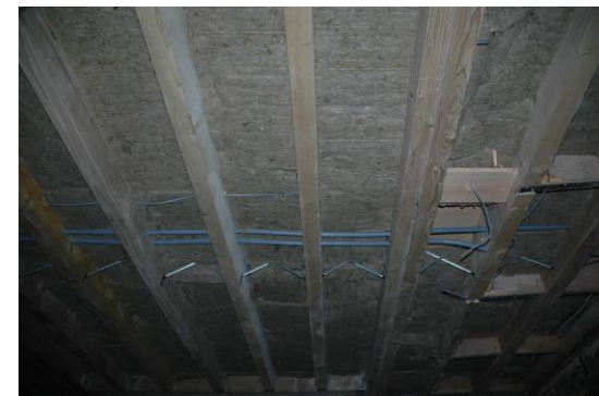
Internal: Photos (a) & (b) Sound insulation (c) Studwork in 2 nd floor flat (hallway outside bedrooms) and (d) insulation, wiring and pipework in the 1 st floor ceiling.
