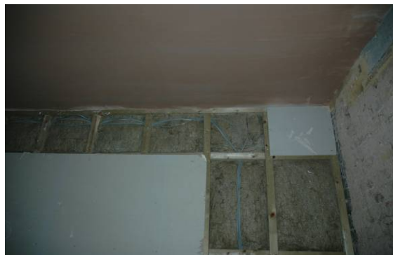
Internal: Photos (a) & (b) Sound insulation (c) Studwork in 2 nd floor flat (hallway outside bedrooms) and (d) insulation, wiring and pipework in the 1 st floor ceiling.
