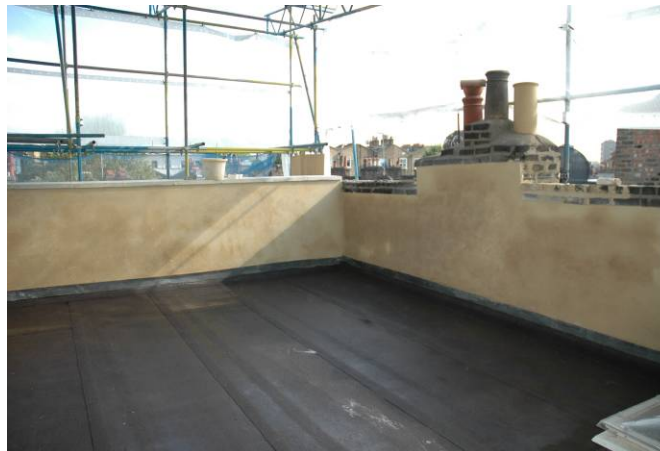
External: Photos (a) & (b) Completed rendering at roof level
